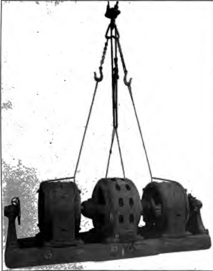
FIG. 29. —Lifting three unit set (wrong way).
